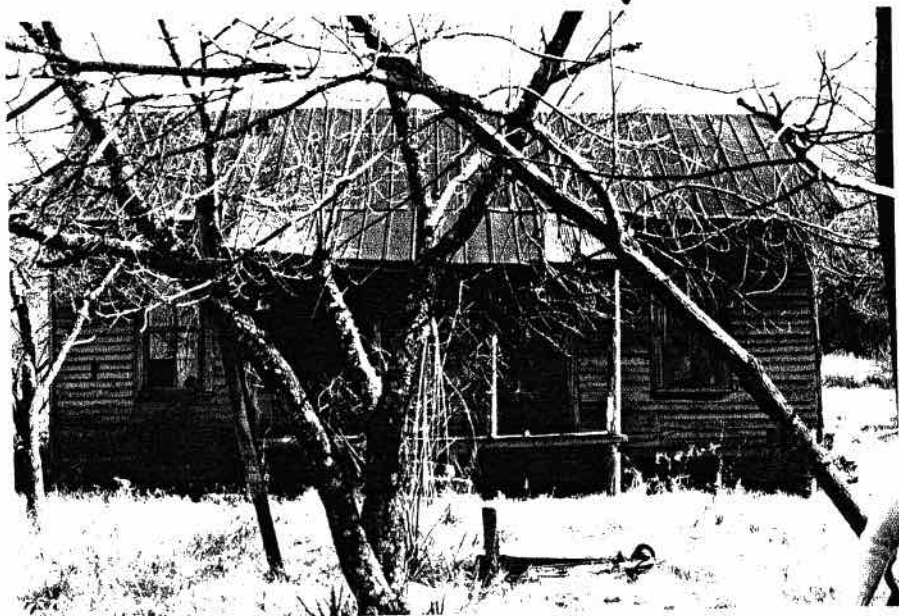
Front of house just before it was torn down. Santa Bottom / Long Hollow.
